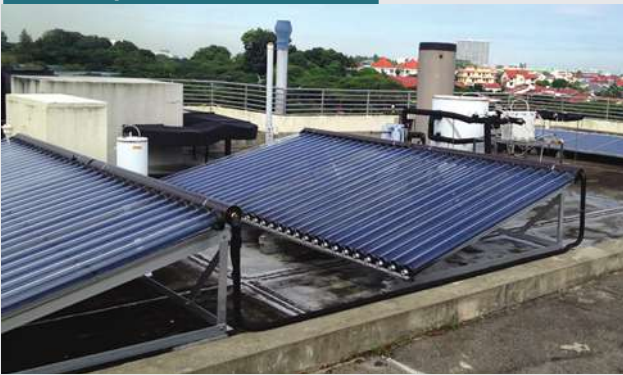
Pilot Rooftop System (@NP)
